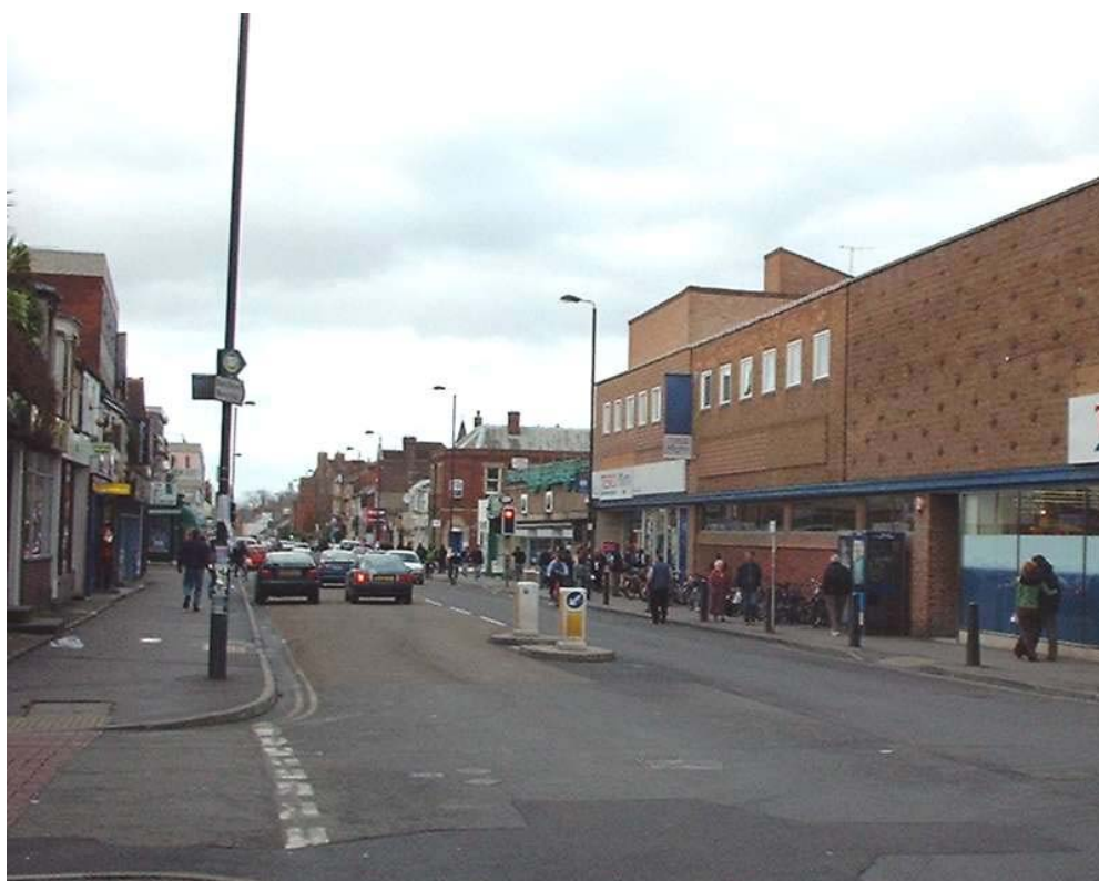
Figure 2 – Cowley Road, Oxford, before treatment
