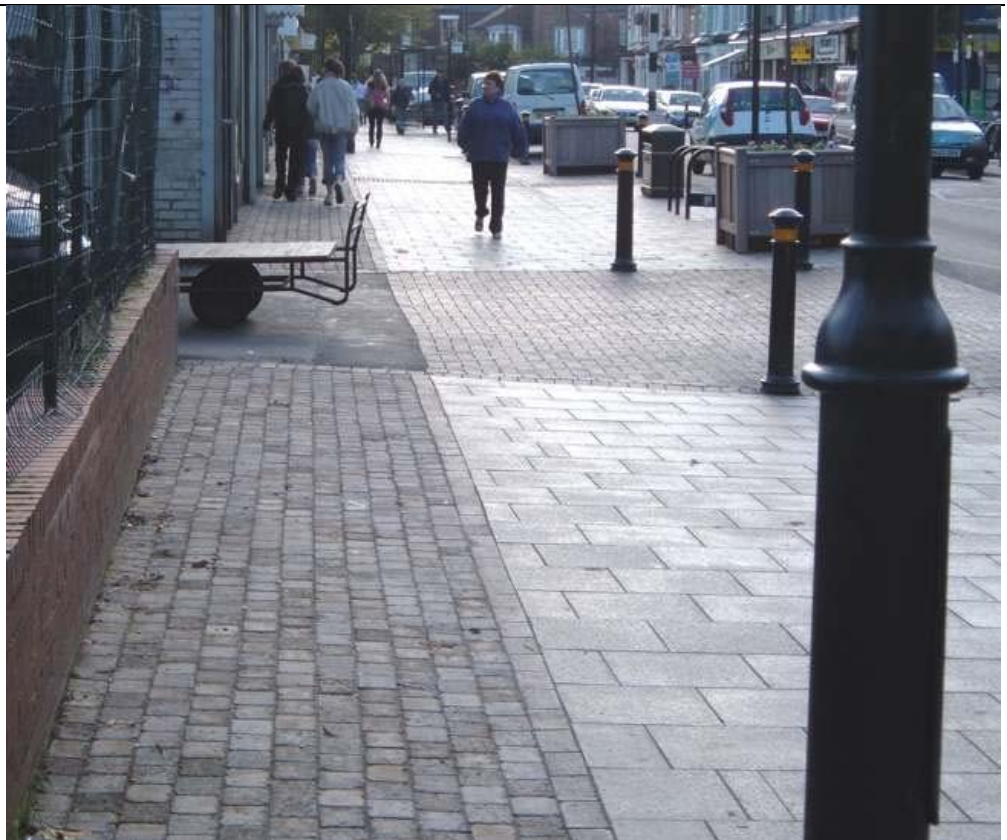
Figure 4 – Newlands Avenue, Hull, after treatment
